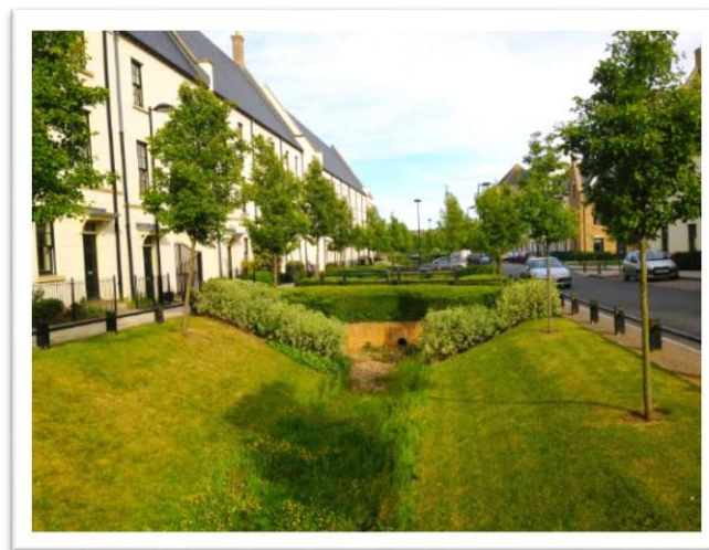
Showing swale drainage system integrated with roads, footpaths and landscape.
